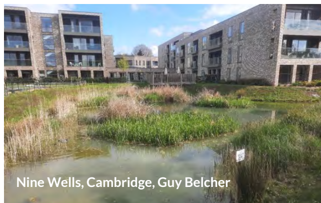
Figure 12 A SuDS feature in a new development
